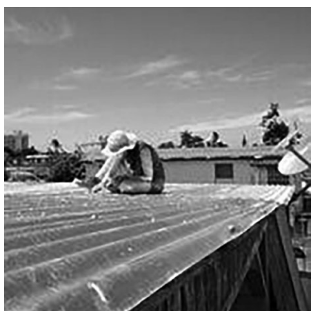
Prof. Llana Barber works on sealing a tin roof.
