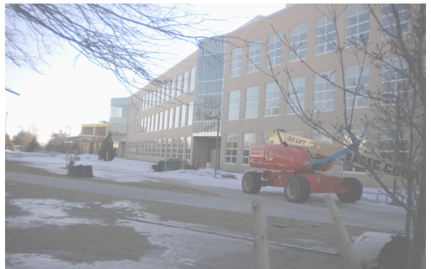
New Academic Building Construction Site
